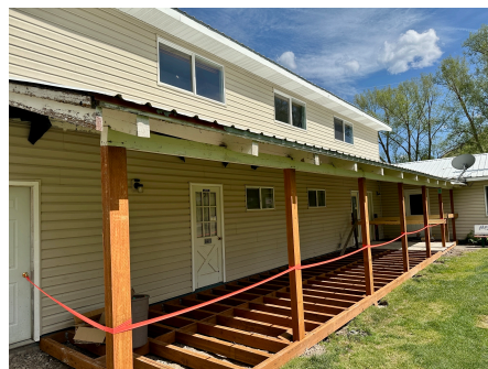
Great Progress! The Patio project in full swing.
